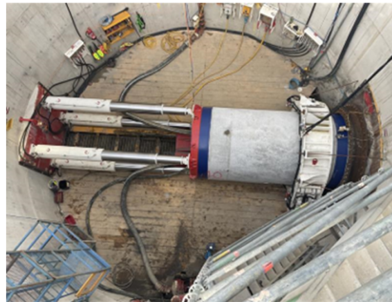
Storm water storage at Ilkley
