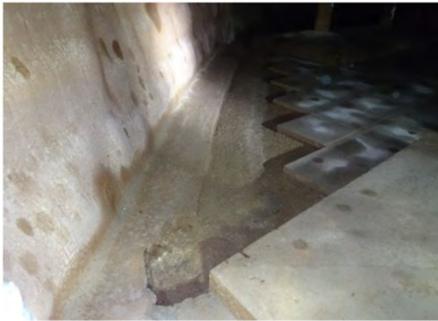
Figure 7.6 Photograph of the floor of Chellow E CWT
