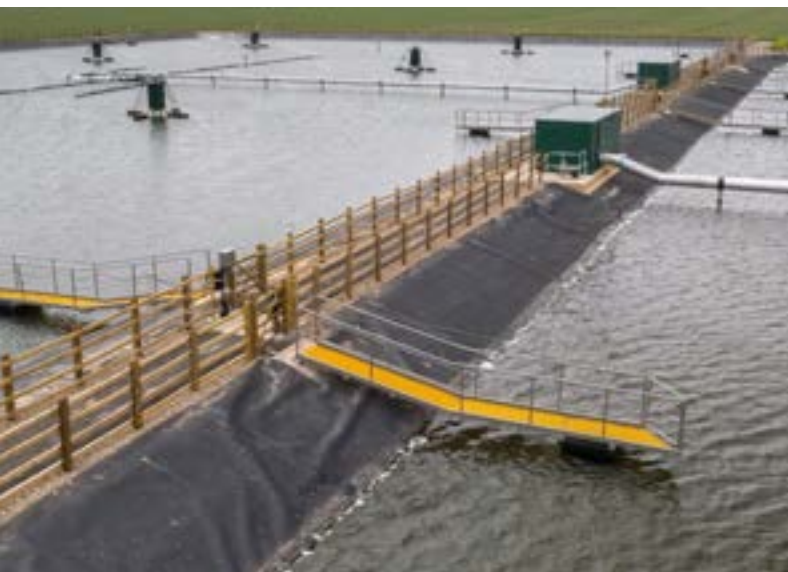
Commissioning the new Aero-Fac® wastewater treatment lagoons near Withernsea
