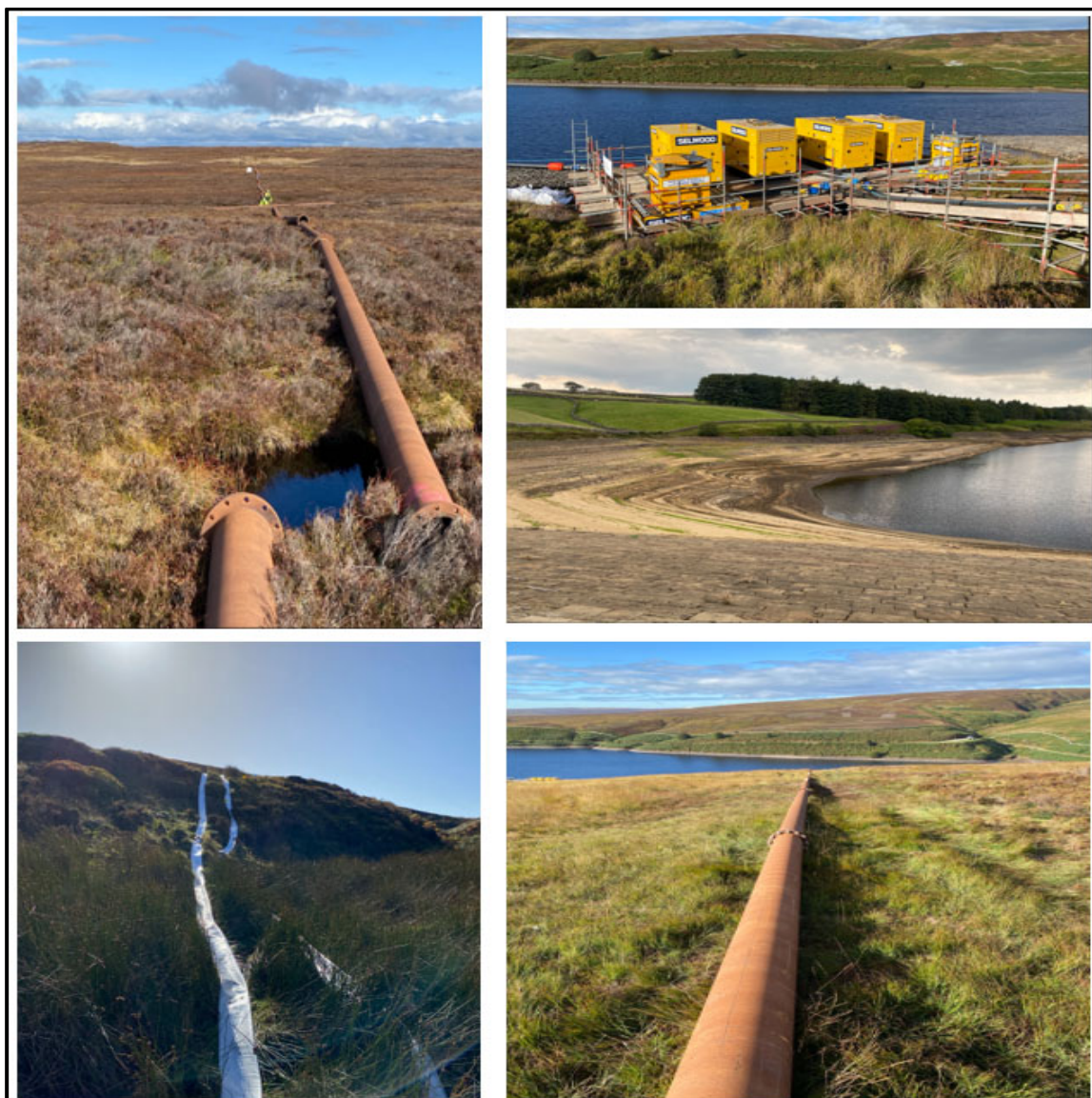
Figure 5 - Images of the emergency scheme to transfer raw water into the Worth Valley
